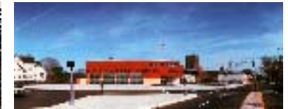
1967-74 Dixwell Fire Station New Haven Connecticut
